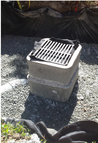
Dry Well systems present an easy to install and sustainable solution for stormwater control.
