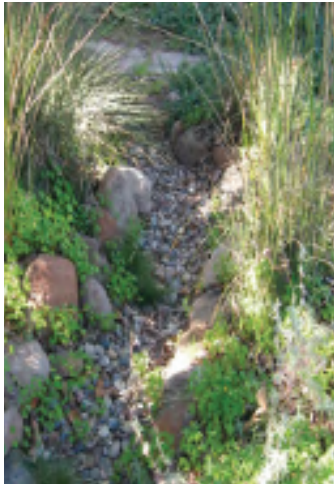
Dry creek infiltrates and conveys runoff.
