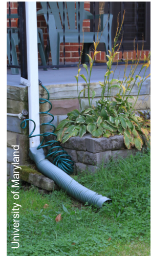
Downspout Connected to Landscape
