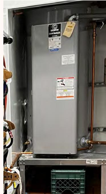
“Designed for use as a recovery heater...NOT recommended for sanitizing water applications”
