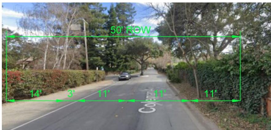
Plate 1 Coleman Avenue West of Berkeley Avenue (County of San Mateo) Looking East
