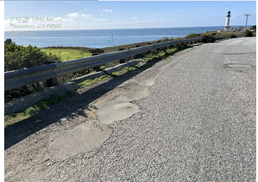
Example of pavement repair areas
