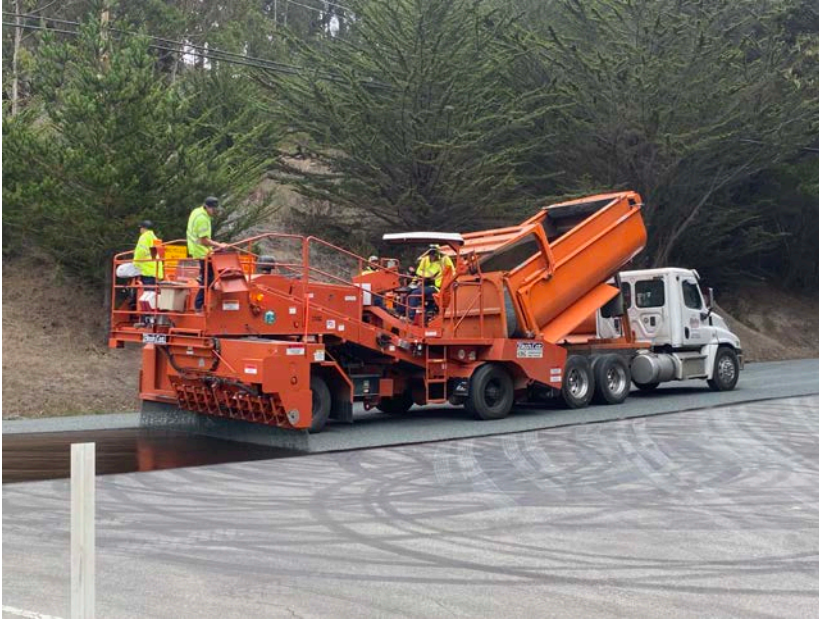
Example of chip seal project in 2022
